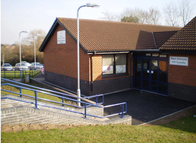
Brackla Community Centre - After
